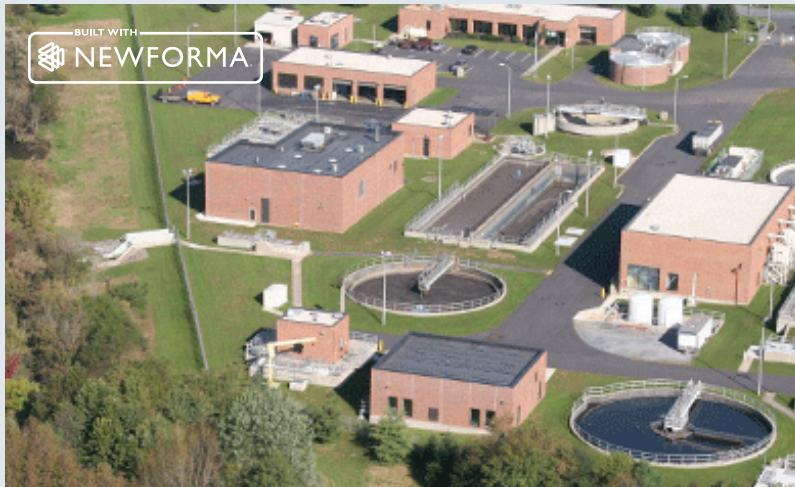
Lititz wastewater treatment facility; Lititz, Pennsylvania
